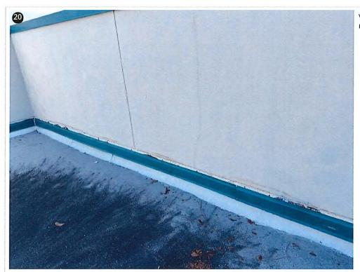
Voids/crack have formed and larger scale repairs will be needed.
