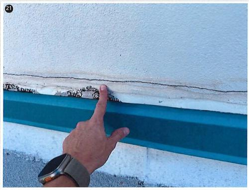
View of large stucco crack forming at the top of the counter flashing, repairs will be needed.
