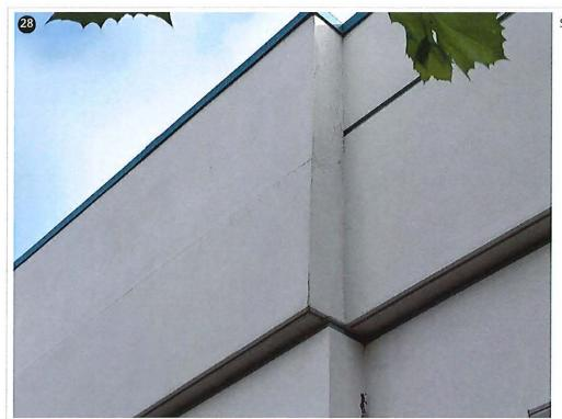
Stucco cracking found near control joints.
