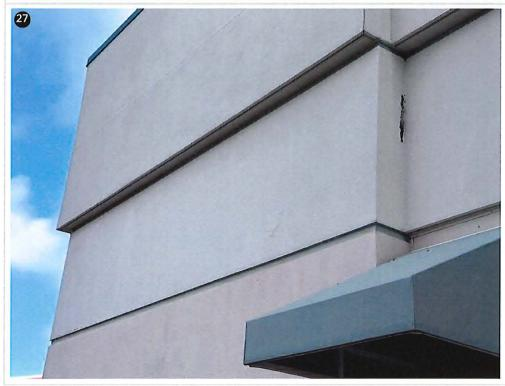
Existing paint has started to bubble/blister in a few locations. I recommend a full building envelope water proofing system which includes stucco repairs.
