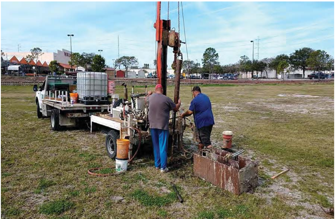
Photograph No. 6: View of soil boring drilling operations.
